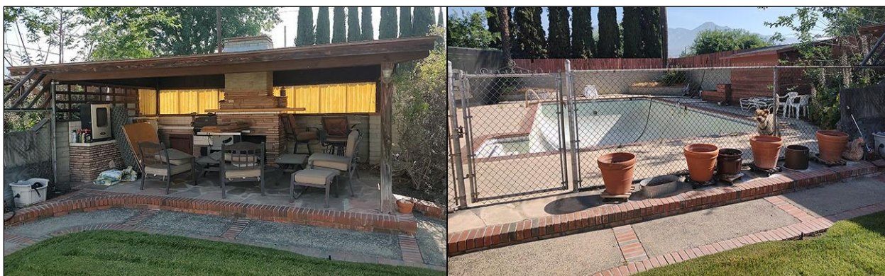
Detached elements. Left : covered patio, view to the east; right : pool (drained), view to the north
