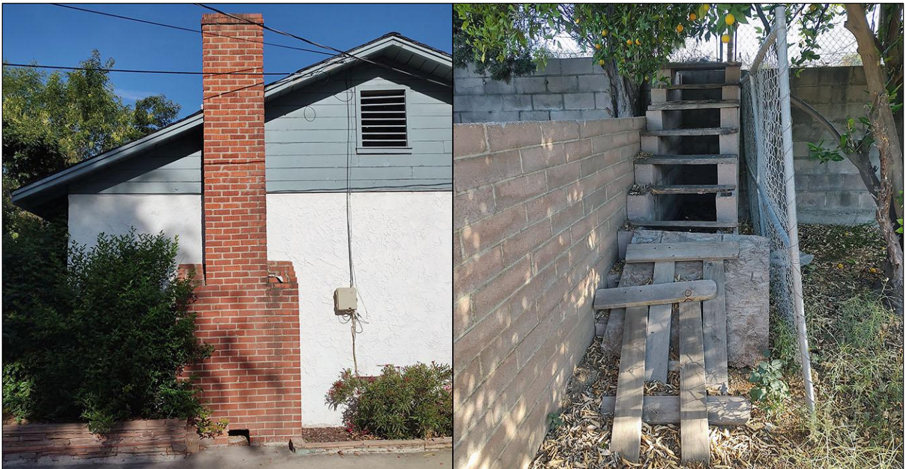
Left: fireplace and chimney; right: stairs to tennis courts on adjacent land
